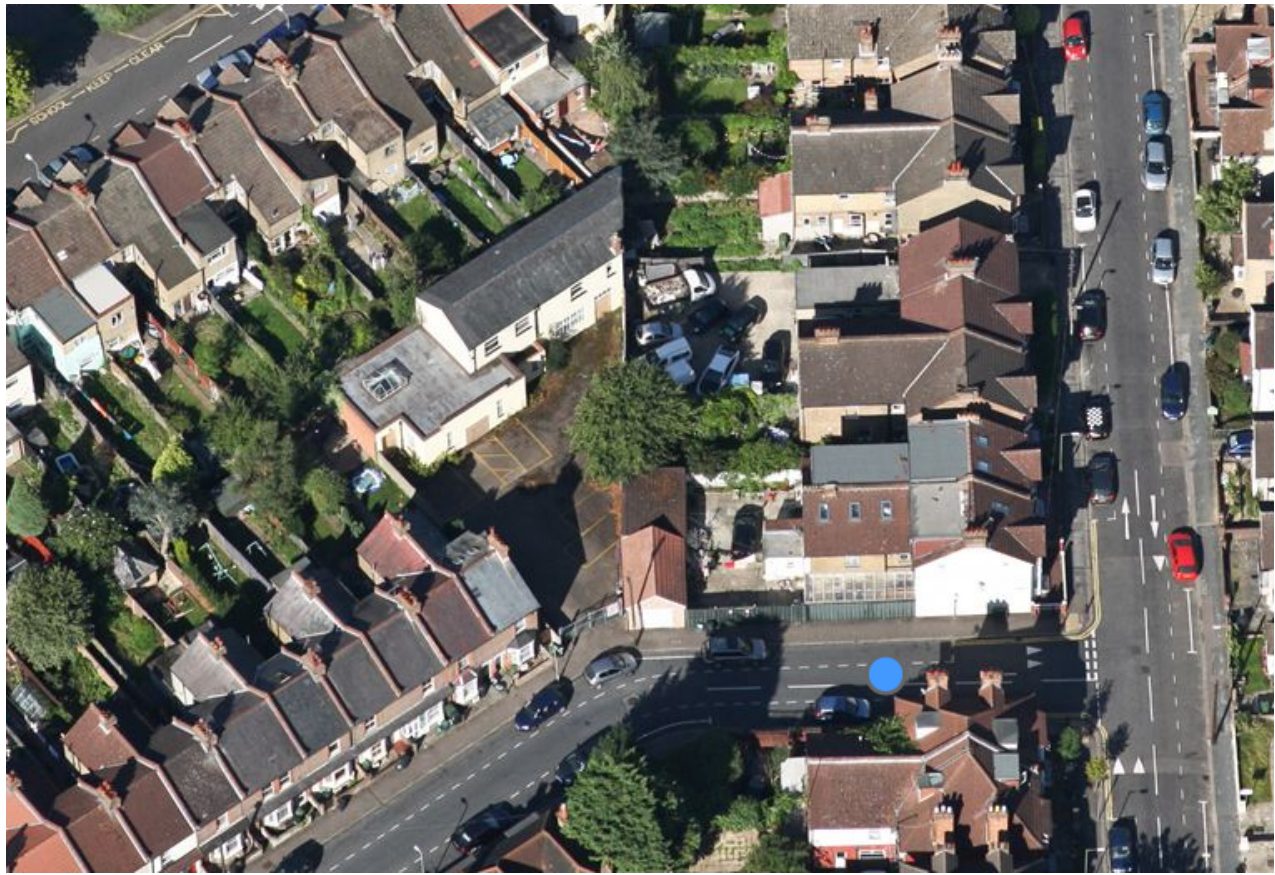
Fig. 1. Aerial view of site.
